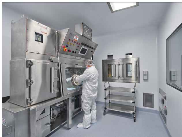
Compounding Room with Isolator
