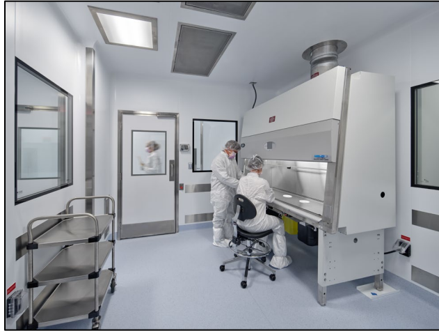
Compounding Room with Biosafety Cabinet
