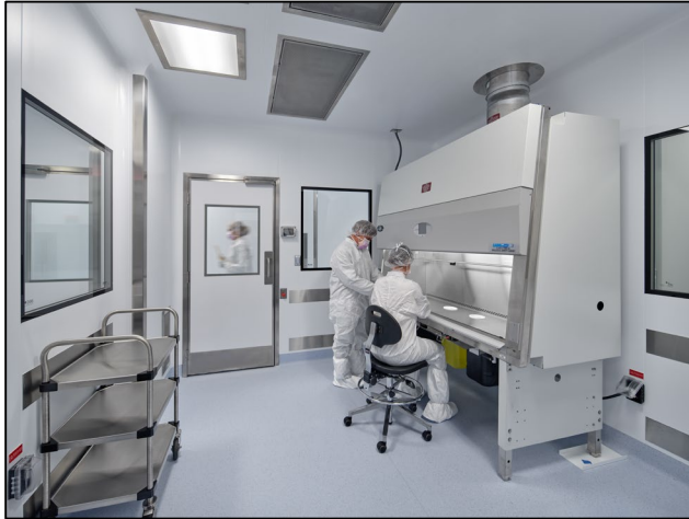
Compounding Room with Biosafety Cabinet
